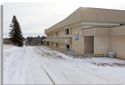
Image – Bus Lane. (East side of school)
