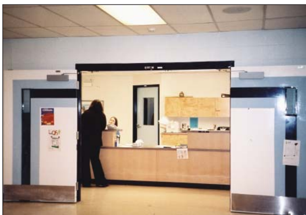
The 2001 BQRP office improvements have improved supervision of the main entrance and lobby and provide a welcoming presence to the general office. The required fire separation resulted in heavier doors.
