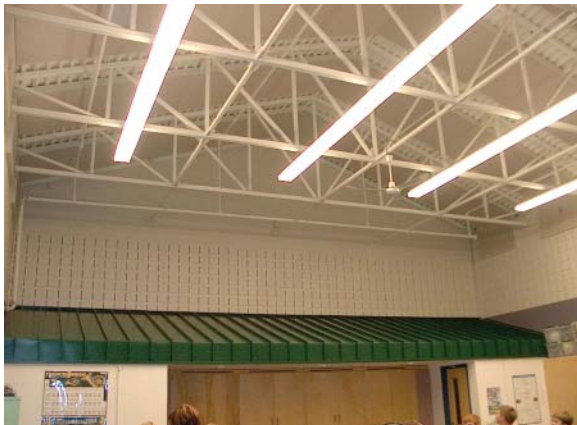
The interior metal sloped roof within the music room should be replaced with more sound absorptive material and could become a mezzanine storage shelf. Storage available for the music room is grossly inadequate.
