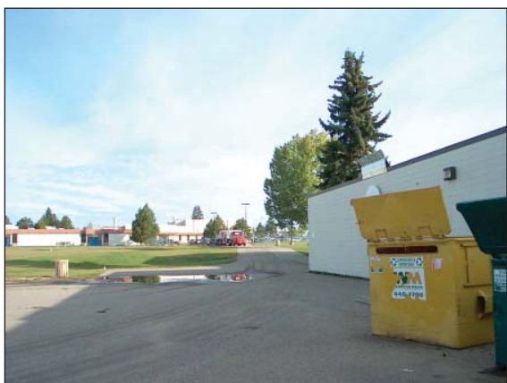
Ponding is evident on the fire lane/access road which is gained through a gated entry from Memorial. When the gate is locked or blocked as photographed above there is no access for emergency or maintenance vehicles.
