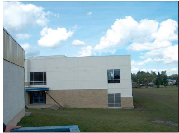
View of the 1999 addition showing an area where run-off causes a muddy slope where there is no sidewalk at a school exit.
