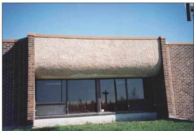
Stone dash stucco soffit is failing and repair is required.
