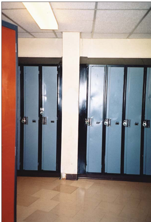
Some student lockers are showing wear and tear. Note the floor settling that requires periodic replacement of floor tiles.
