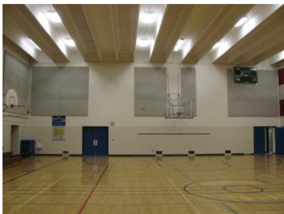
The fabric panels in the large gym are damaged and require replacement.
