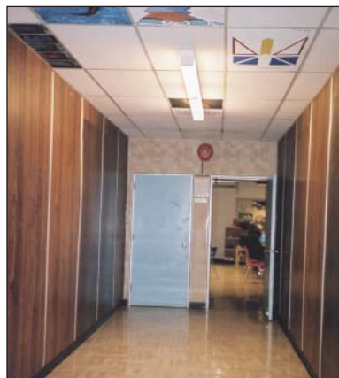
The five locations where corridors lead to twin classrooms, four of them joined, additional means of egress is provided through adjacent classrooms. Same wall finishes may not meet flame-spread ratings.
