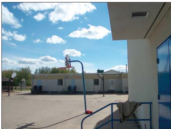
View of the paved play area behind the school. Poor surface drainage from the bus lane results in flooding of the play area beyond.
