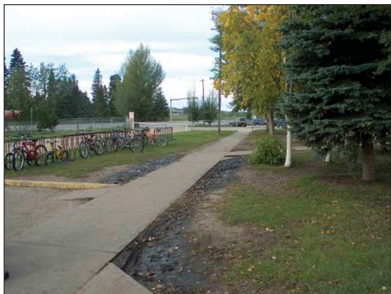
The main entrance sidewalk and adjacent grounds require re-grading to prevent ponding and ice build-up.
