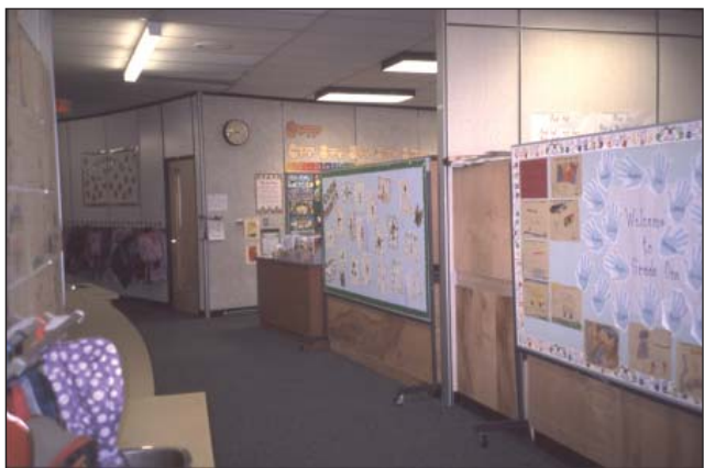
Formerly an open classroom plan attempts have been made to gain acoustic privacy with the placement of millwork which also defines classroom boundaries.
